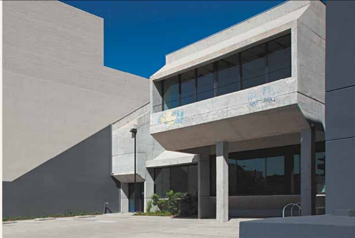
Previous page: Clare Cousins in the meeting room at the Blackwood Street Bunker. Photograph by Daniel Aulsebrook. Above: raw beauty of The Blackwood Street Bunker. Photograph by Lisbeth Grosmann. Opposite: breeze blocks and framed views in 'the Bunker'. Photograph by Lisbeth Grosmann.
